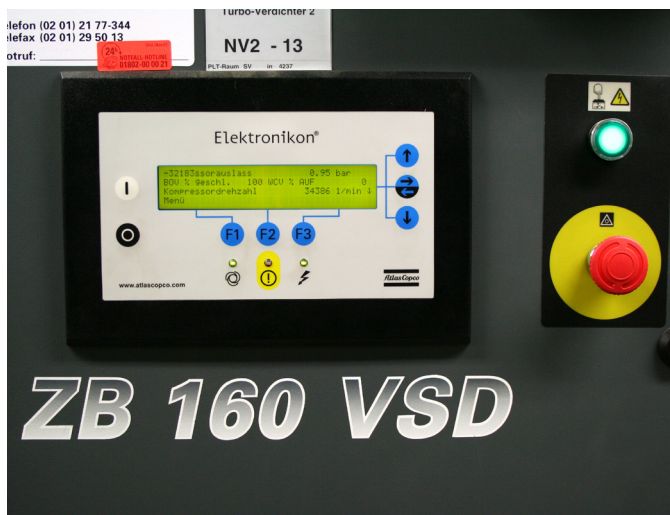
Fig. 4: The four speed-controlled (“VSD”) centrifugal compressors are controlled using the ES 130T higher level control unit, optimized for energy. This separate control unit can also be retrofitted for existing installations.
