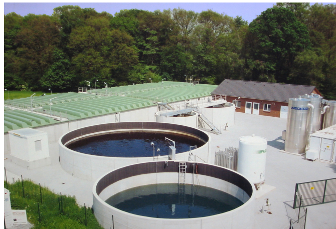
Fig. 1: The seepage water waste water treatment plant at the Münster waste management center
