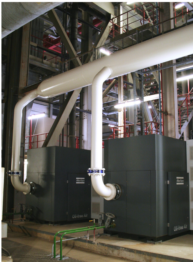
Fig. 4: The compressed air is routed over the white distributing main into the absorber.
