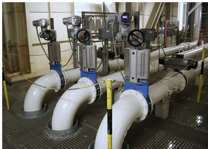
Fig. 3: Distributor for three absorbers where the flue gas is desulphurized. This is where the sulfuric acid components of the gas are combined with the alkali portions of the added lime wash. The result is gypsum and clean exhaust air.
